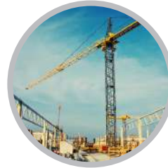
Cantiere Building site
